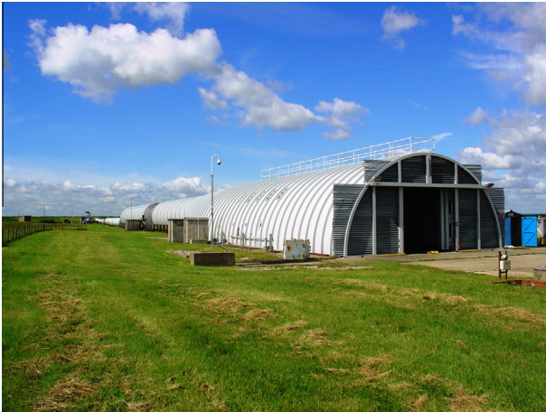
Fig. 1. Air blast tunnel – entire structure.
