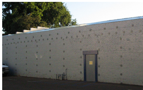
(a) External view showing extensive through-wall anchorage of internal steel strong backs installed for increased out-of-plane wall stability
