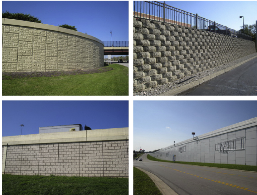
Fig. 1. Several constructed MSE wall examples.
