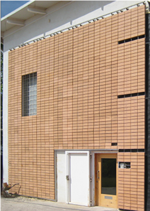
Fig. 1. External TCT curtain wall ( www.flexbrick.es ).
