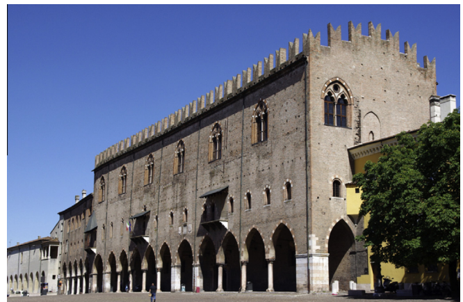
Fig. 1. Picture of Palazzo del Capitano in its current state taken from Piazza Sordello .
