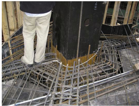
Fig. 1. Configuration of the ring-beam connection.
