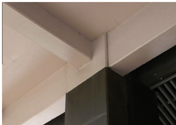
Fig. 1. Interior beam–column joint with smaller-size transverse beam.
