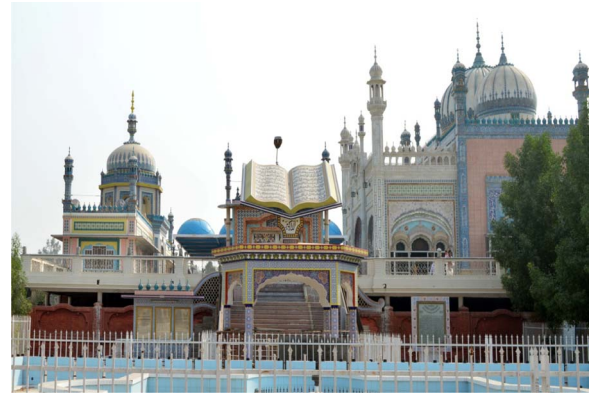
Figure 1 View of the modified Bhong Mosque (Picture is taken by the Author).
