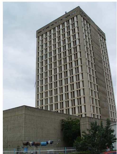
Fig. 1 Rilindja Printing House Tower. Original design (Photo: Petrit Rrahmani).
