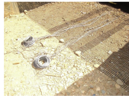
(b) Installation of one of the instrumented reinforcement layers
