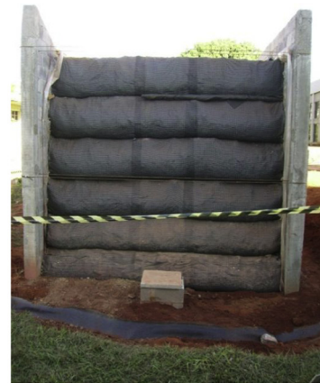
(c) Wall face at the end of construction.
