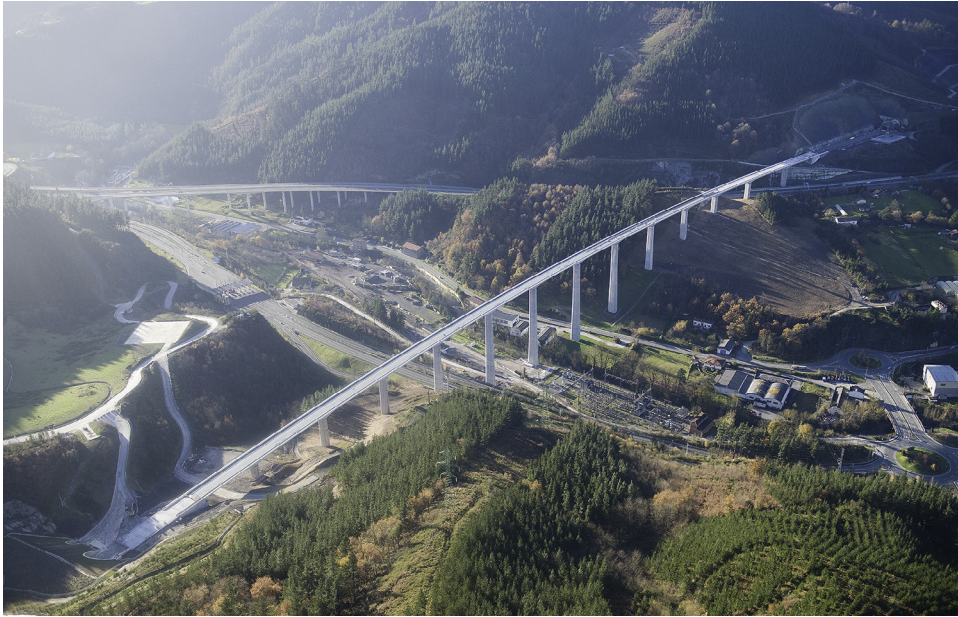
Figure 1. Finished River Deba Viaduct.
