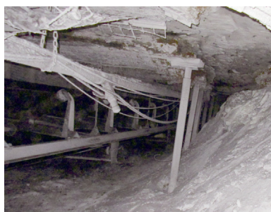
Fig. 2. Pillar sloughage and extended roof span.
