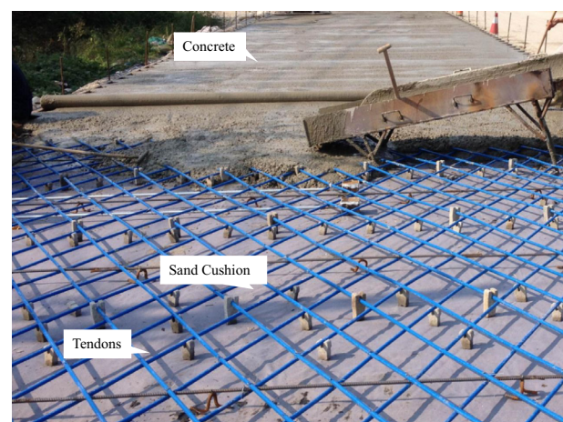
Fig. 1. Construction of CTCP.
