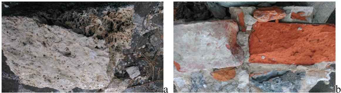
**Fig. 2.** In situ materials: calcareous stone masonry (a) and clay-brick masonry (b).
