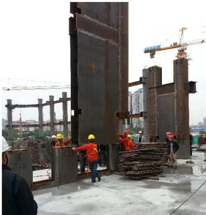
(c) Installation of composite shear wall
