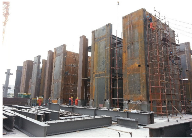
(b) Photo of building site
