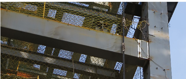
Fig. 2. Beam with side plates.
