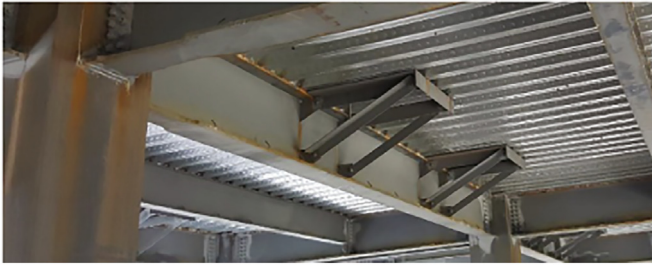
Fig. 1. Beam with lateral bracing.
