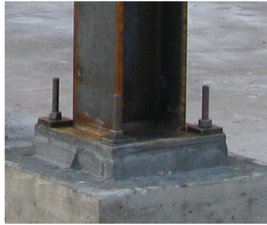
Fig. 1. A typical exposed, unstiffened column base connection [18]
