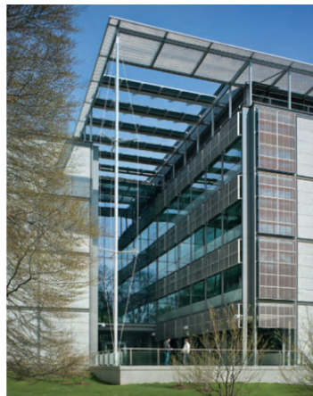
(b) Stiffened column in Princeton, U.S.A
