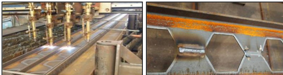
Fig. 2. Fabrication of the test members [2].
