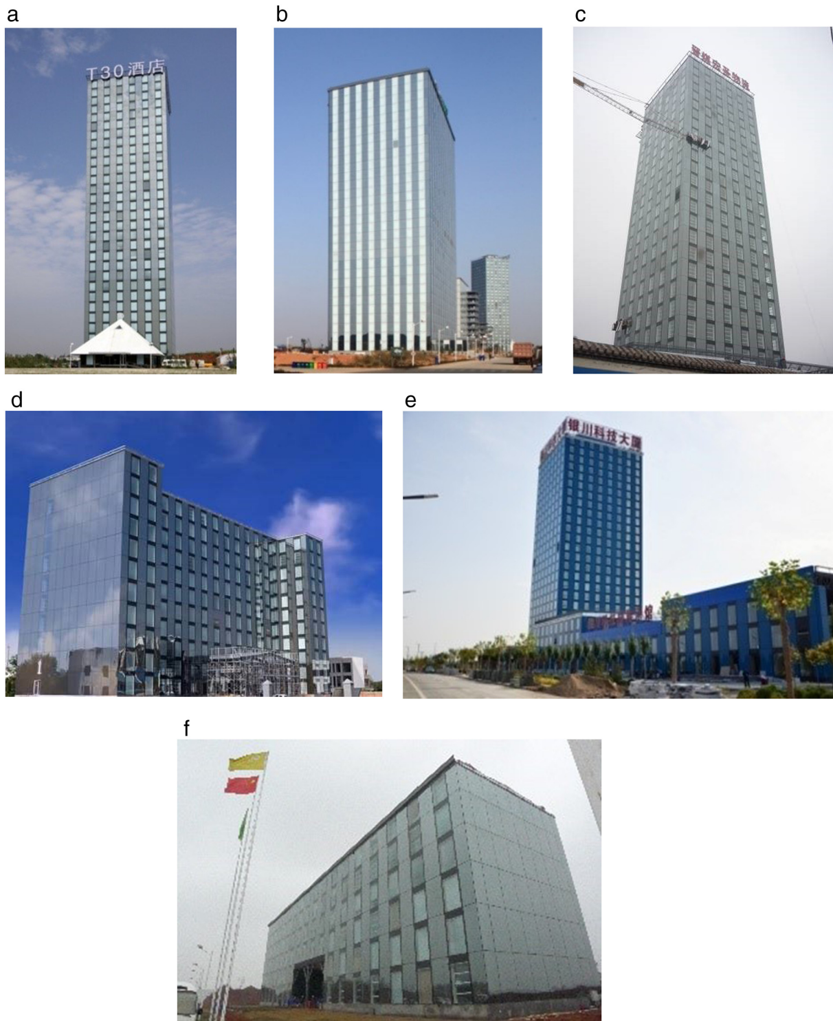
Fig. 1. Modular-prefabricated high-rise steel frame structures with diagonal braces. (a) A 30-story hotel. (b) A 30-story apartment. (c) A 26-story multiple-use building. (d) An 11-story office building. (e) A 25-story technology mansion. (f) A 6-story office building.
