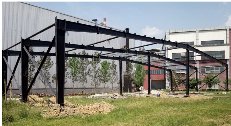
(b) frame on site
