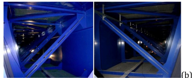
Fig. 1. Sesia viaduct: (a) general view of the spans and (b) interior view of the double-box girder.
