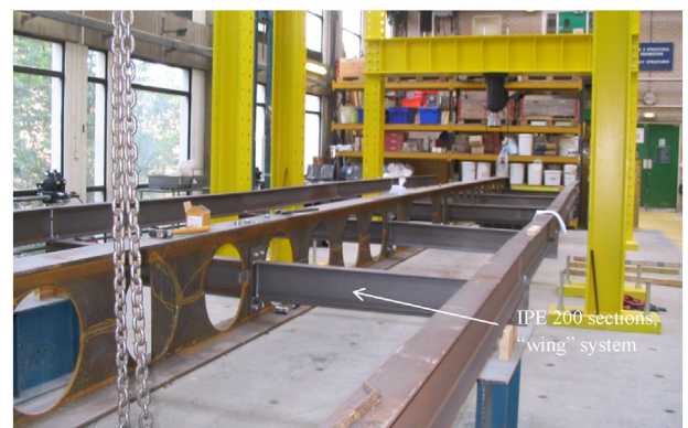
Fig. 3. “Wing” system used to support wet concrete slab weight.
