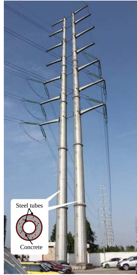
Fig. 1. CFDST electric poles in Hangzhou, China.
