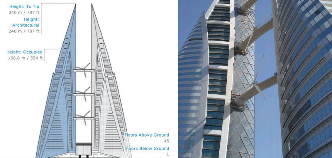
Fig. 1. Wind turbines integrated in between the Bahrain World Trade Center Towers. ( http://www.skyscrapercenter.com/building/bahrain-world-trade-center-1/998 ).
