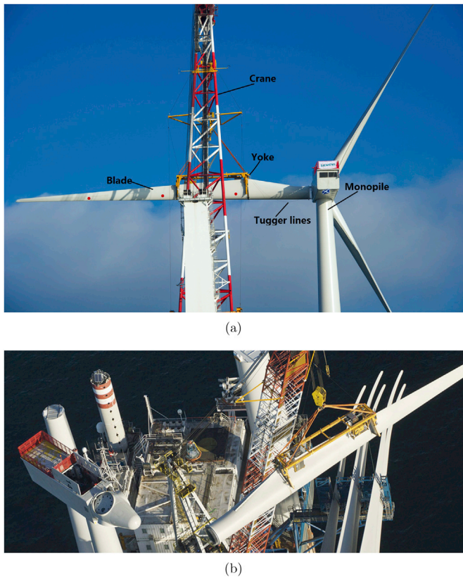
Fig. 1. Image of a horizontal single blade mounting on offshore wind turbines (a) side view (Image source: Siemens Wind Power GmbH) (b) top view (Image source: A2SEA A/S).
