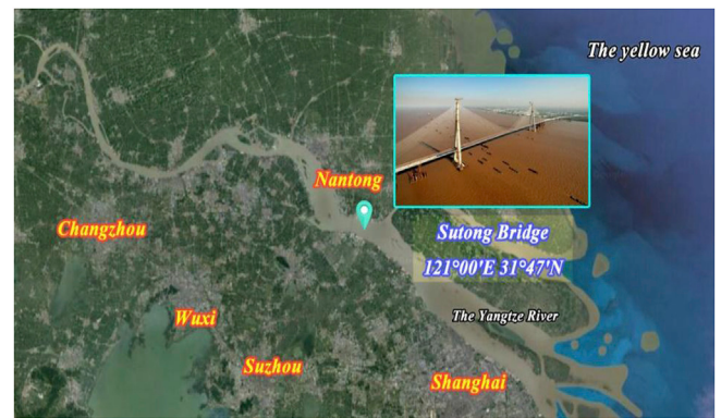
Fig. 1. Location of Sutong cable-stayed Bridge.
