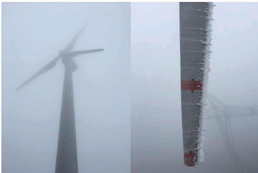
Fig. 1. 300 kW wind turbine and overnight ice accretion on its blade.
