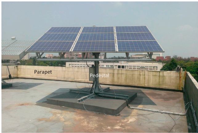
Fig. 1. Photograph of solar trackers on a flat-roofed building in the campus of National Central University, Taiwan.
