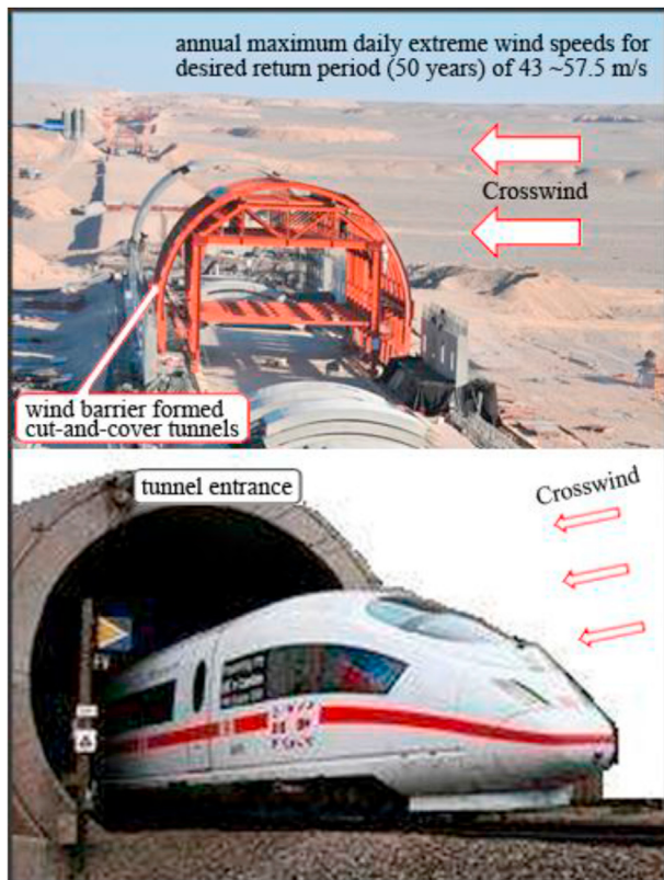
Fig. 2. Wind barrier formed cut-and-cover tunnels.
