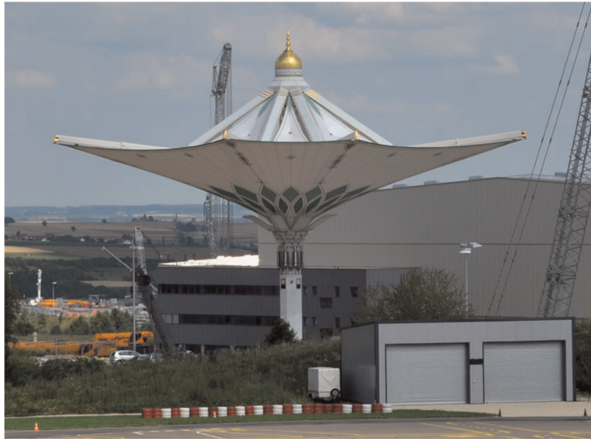
Fig. 1. Prototype of a 53 m umbrella, SL-Rasch GmbH at the factory site of Liebherr.
