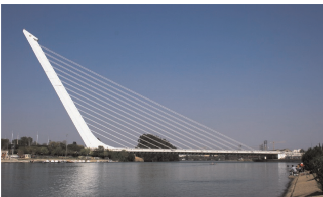
Fig. 1. The Alamillo Bridge in Spain.
