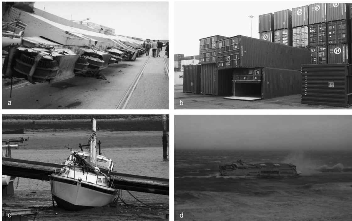
Fig. 1. Examples of wind-induced risks and damages in port areas: collapse of a harbour crane (a); containers overturning (b); collapse of lighting tower, fallen over a boat (c); the ferry boat Fantastic entering the Port of Genoa during a sea storm on 30th October, 2008 (d).
