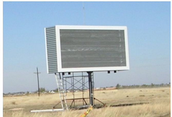
Fig. 1. A prototype rectangular sign structure subjected to monitoring.
