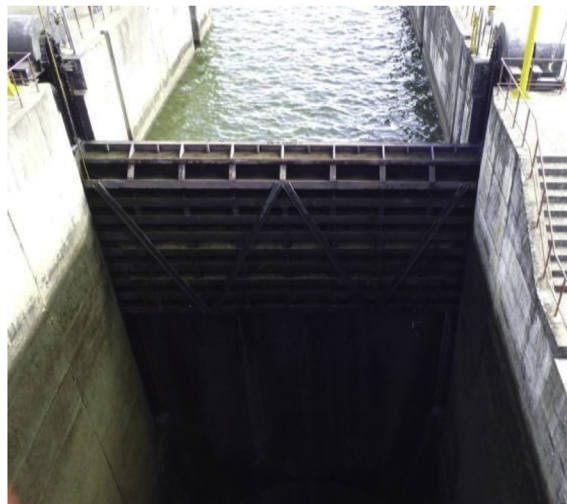
Fig. 2. Upstream lock gate in closed position.
