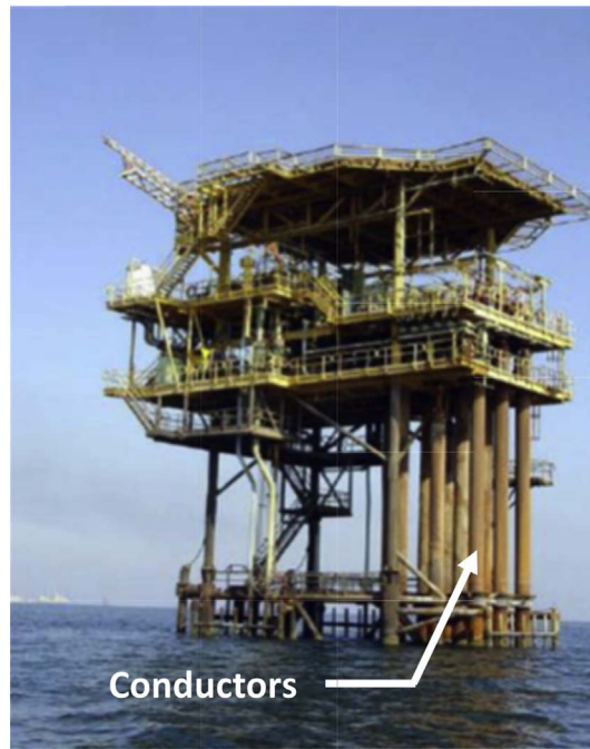
Fig. 1. Shallow water jacket platform in the Persian Gulf, showing typical conductor arrangement [4].
