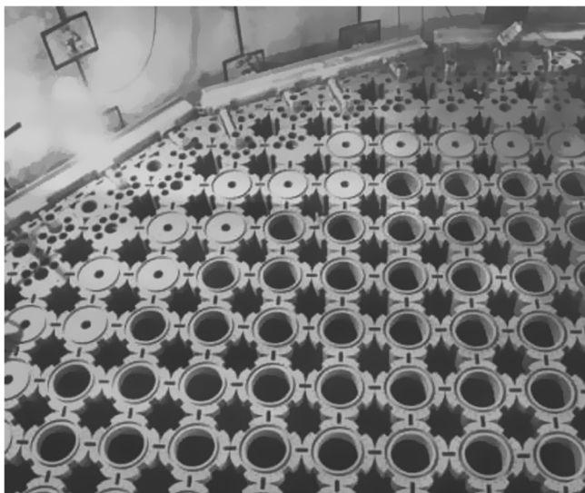
Fig. 1. The lattice of graphite bricks comprising the core in an advanced gas-cooled reactor.
