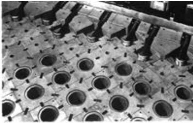
Fig. 1. Shows arrangement of bricks in reactor core.
