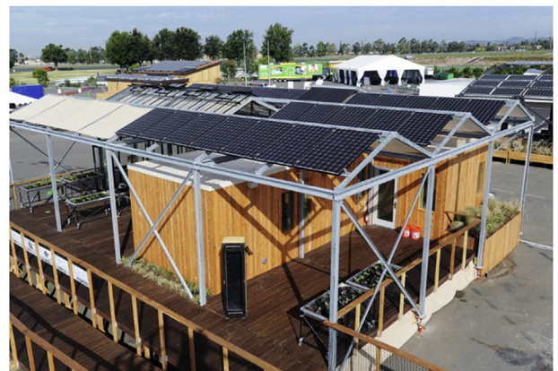
Fig. 1. The GRoW Home by day at the competition site in Irvine, CA. Photos by Thomas Kelsey/U.S. Department of Energy Solar Decathlon.
