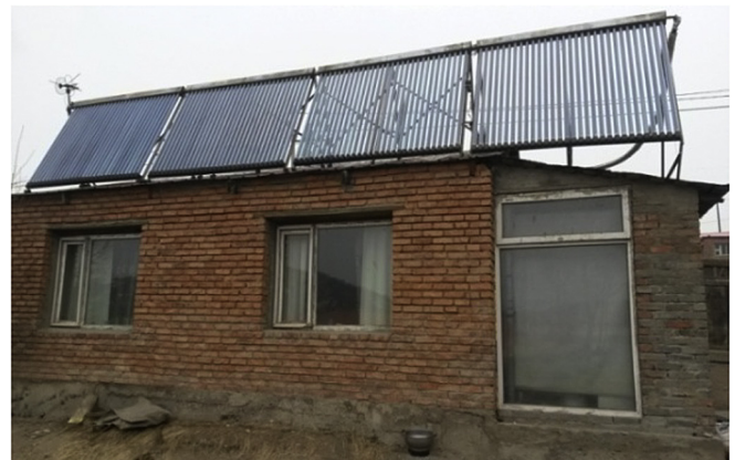
Fig. 1. Overview of the measurement house.
