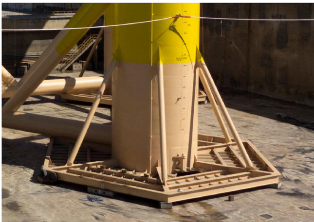
Fig. 1. Detail of a WindFloat prototype column. Photo courtesy of Principle Power.
