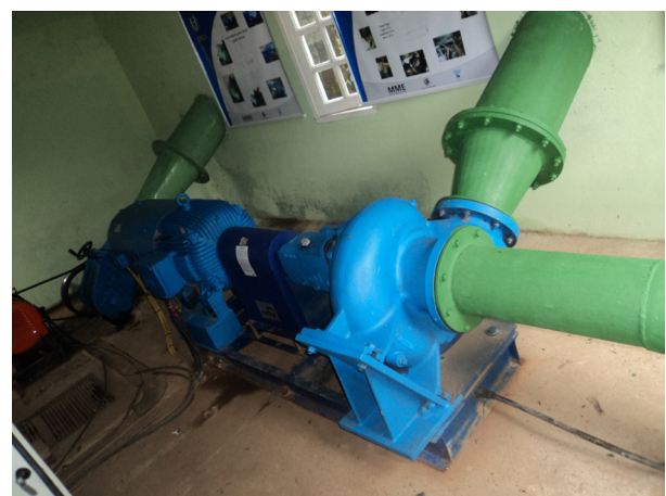
Fig. 2. Pump as Turbine/Induction Generator group.
