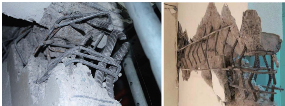
Fig. 2. Low-cycle fatigue failure due to rupture of the main bars at the end of RC walls, Chile [6,7].
