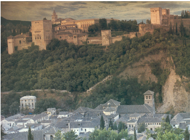
Fig. 1. View of San Pedro Cliff.
