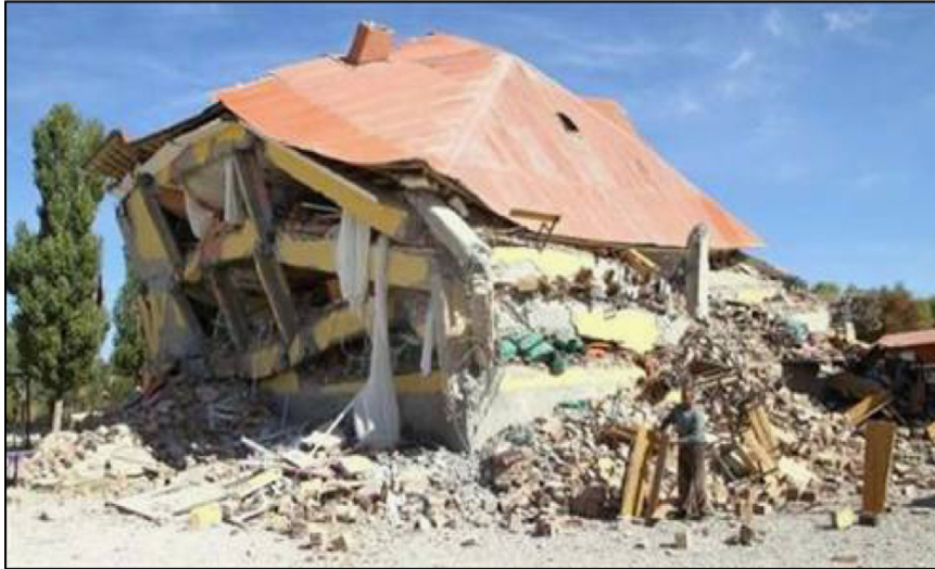
Fig. 1. Gedikbulak primary school after the M_w=7.0 Van-Turkey Earthquake on 23 October 2011.
