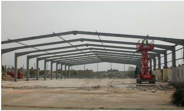
Fig. 1. Hot-rolled steel portal frame.
