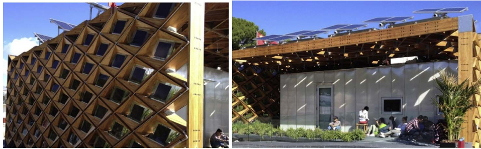
Fig. 1. The Eco-House prototype exhibited at SDE 2012. BIPV systems are used in the façade and BAPV on the roof.
