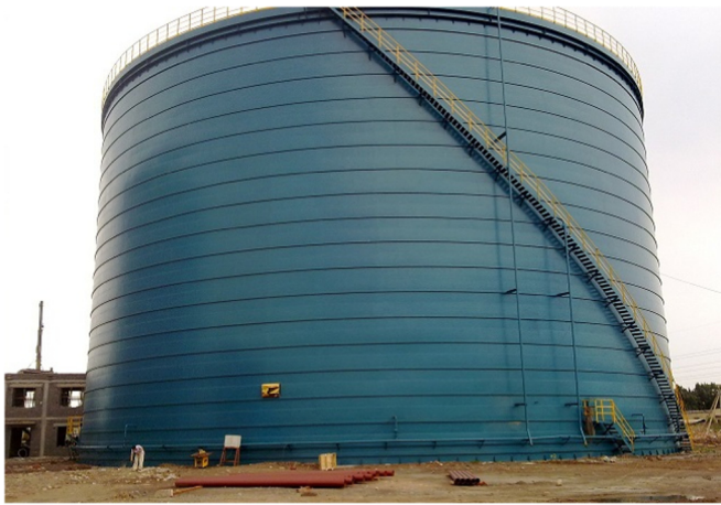
Fig. 1. A typical ground-supported circular steel silo with a capacity of 57,000 m 3 .
