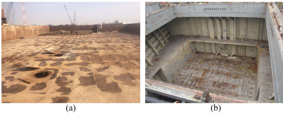
Fig. 1. (a) Deformed deck plate of a landing craft due to the overloaded trailers, (b) deformed structure of tank top of a general cargo ship.
