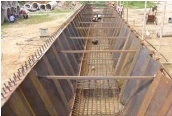
Fig. 3. Inclined bridge girders with corrugated steel webs.
